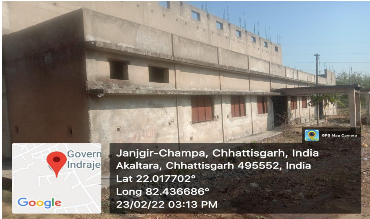
INDOOR STADIUM (UNDER-CONSTRUCTION)
